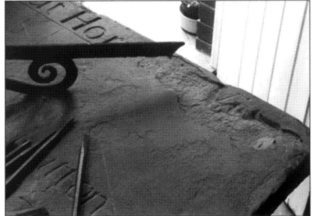
Fig.7. The top right-hand edge of the E dial plate, showing deep decay and the remains of the original motto.
