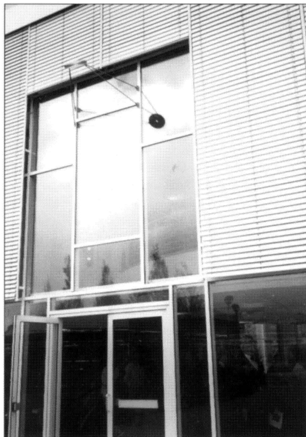
Fig.2. The gnomon showing the supporting struts, with the shadow indicating its shape. The blinds on the side windows are an energy conservation system, rising and lowering, opening and tilting as the sun goes in and out.
