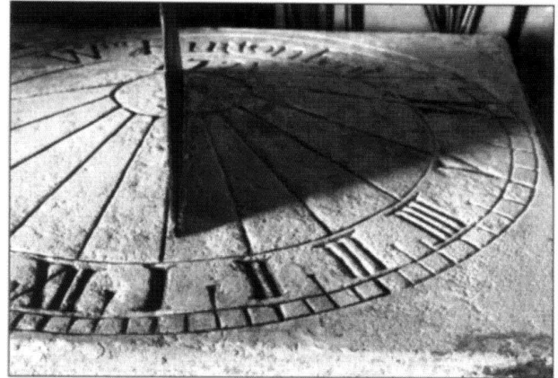
Fig.3. The S dial during restoration; some of the lines and numerals have been coloured in matt grey.
